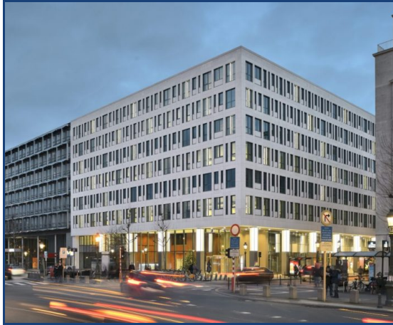
Arts 58 Bureaux locaux location bruxelles facade
